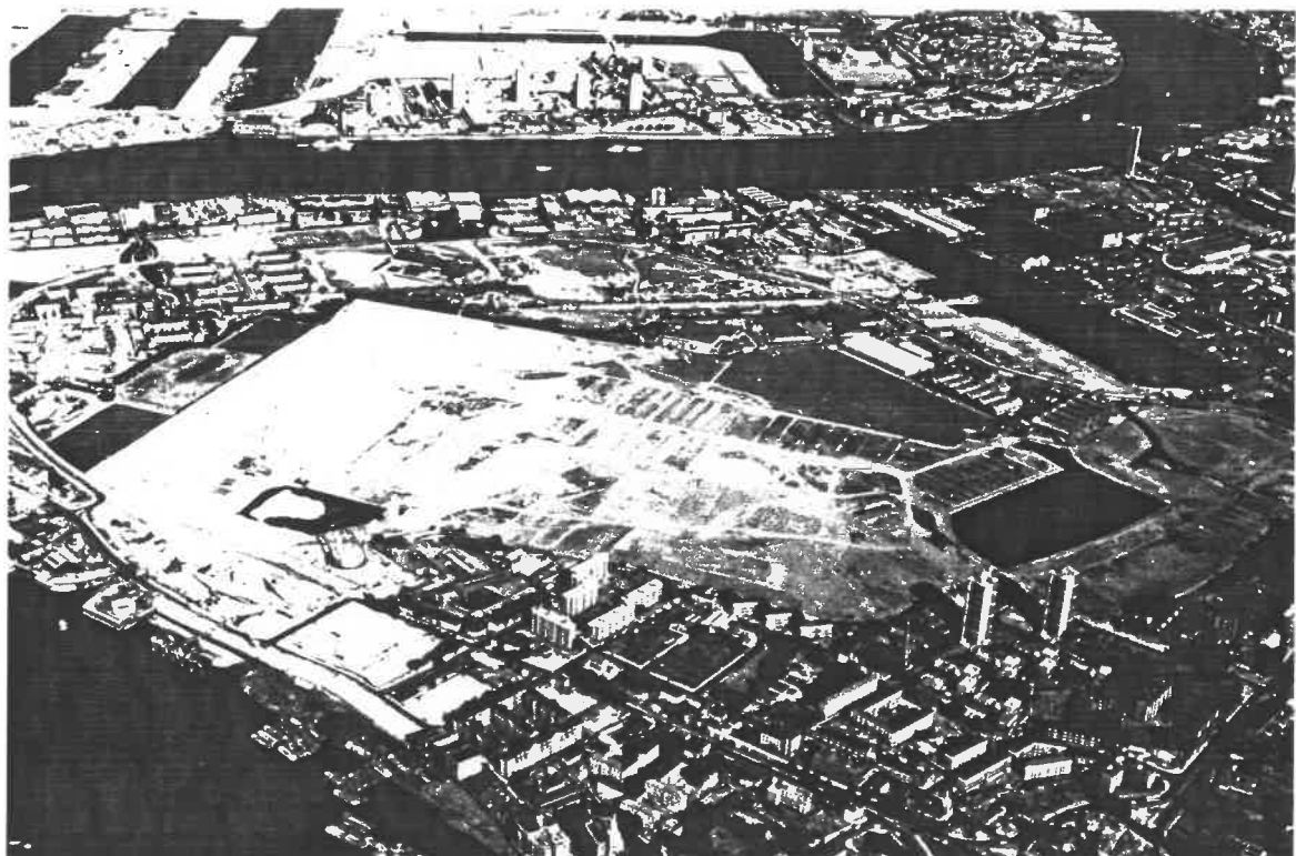
FIGURE 3 - SURREY COMMERCIAL DOCKS (AFTER FILLING)
