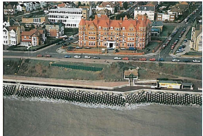
Clacton - tunnel line about 15m from cliff edge (courtesy A F Howland Associates).
