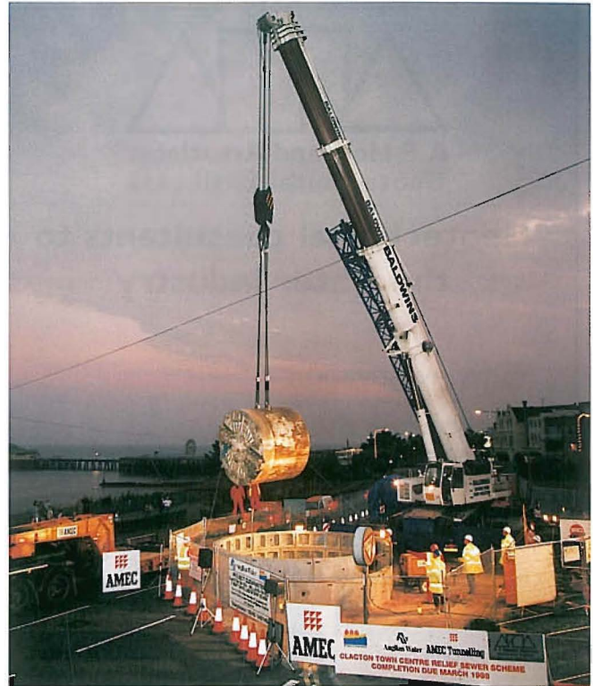
Clacton - recovery of Lovat 101 machine (courtesy Anglian Water Services Ltd).
