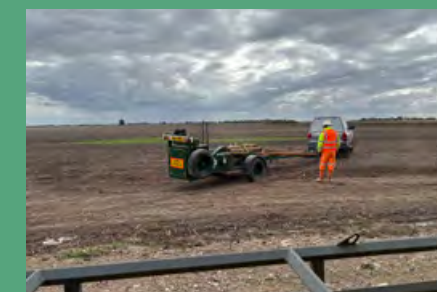
Trenchless Construction Services
